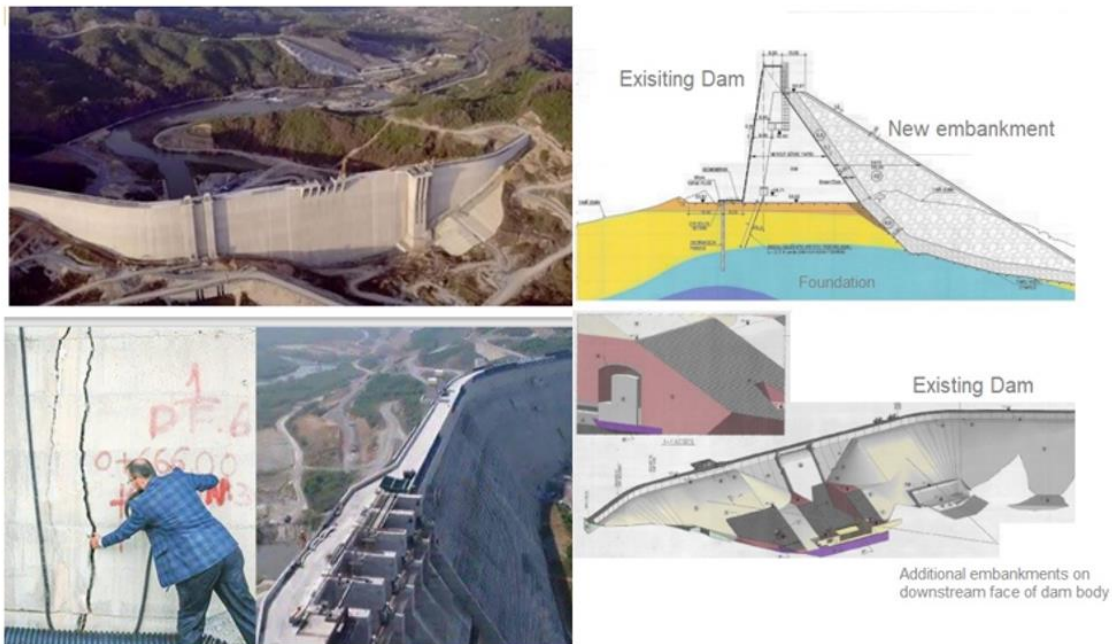
Figure 9. Cracks in the Melen Dam Body and its strengthening project
