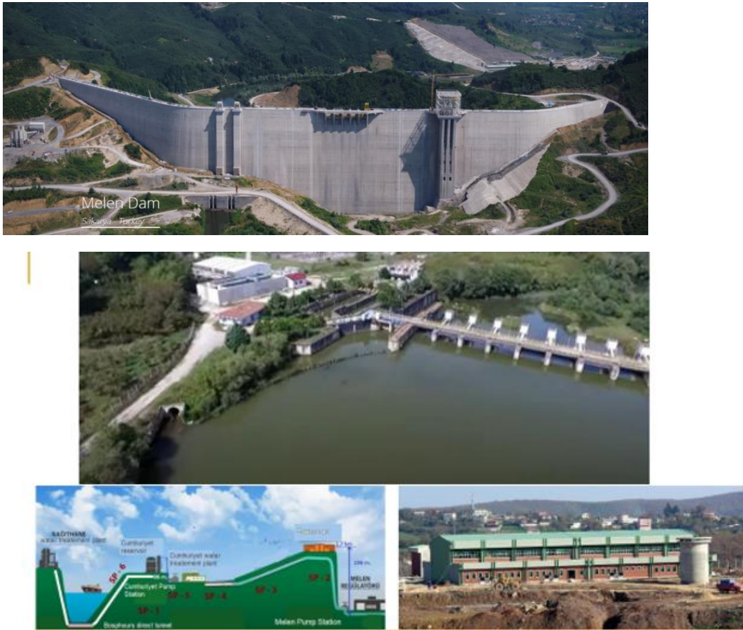
Figure 10. Melen Dam, Melen Regulator and Pumping station
